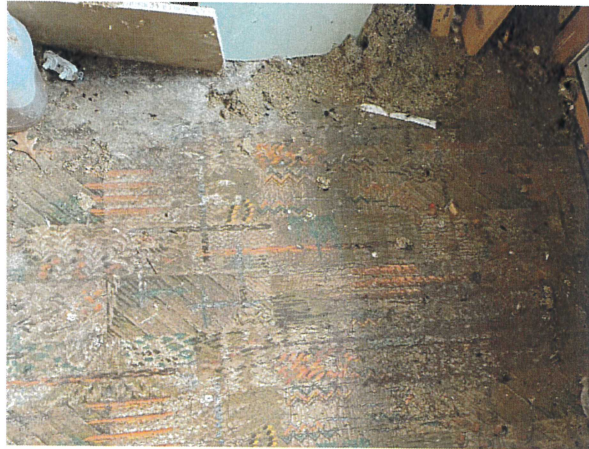
FAI-310-090223-001, 002, 003 None Detected, Multi-colored Vinyl Sheet Flooring
