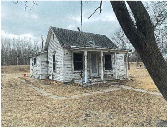
Northeast exterior elevation viewing southwest
