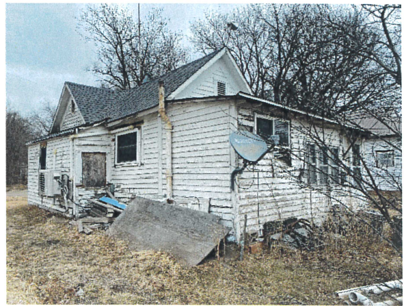
Southwest exterior elevation viewing northeast
