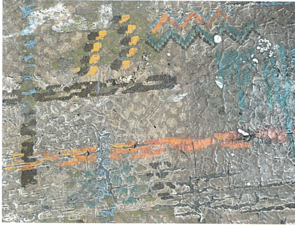
FAI-310-090223-001, 002, 003 None Detected, Multi-colored Vinyl Sheet Flooring
