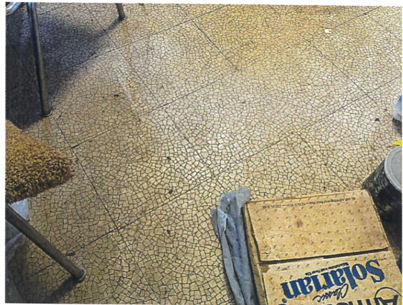
FAI-322-130223-004, 005, 006 2% / 2% , 12" x 12" Brown Vinyl Floor Tile / Black Mastic
