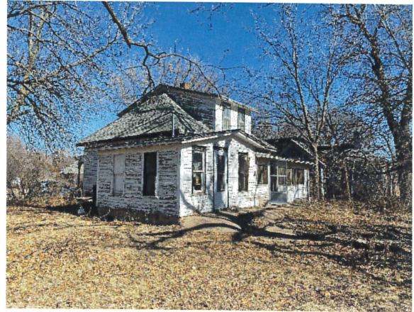
Southwest exterior elevation viewing northeast
