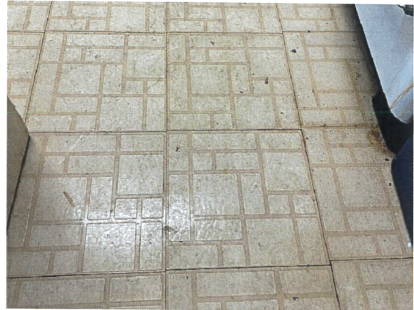
FAI-322-130223-001, 002, 003 None Detected, 12" x 12" Tan Vinyl Floor Tile
