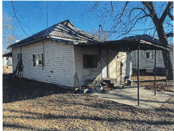
Southwest exterior elevation viewing northeast
