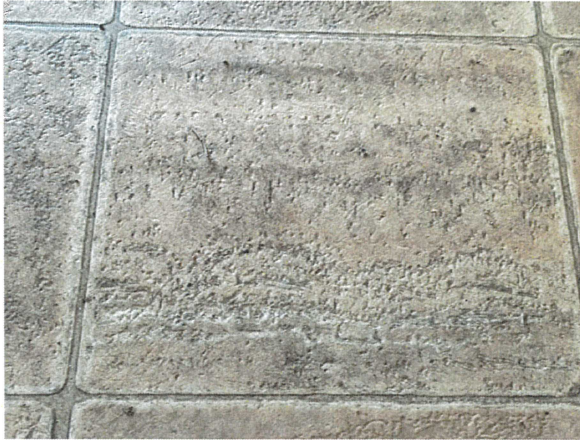
FAI-121-100223-001, 002, 003 None Detected, Brown Vinyl Sheet Flooring
