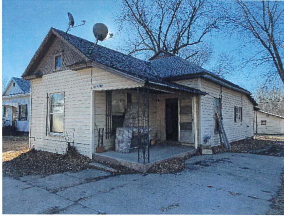
Northwest exterior elevation viewing southeast
