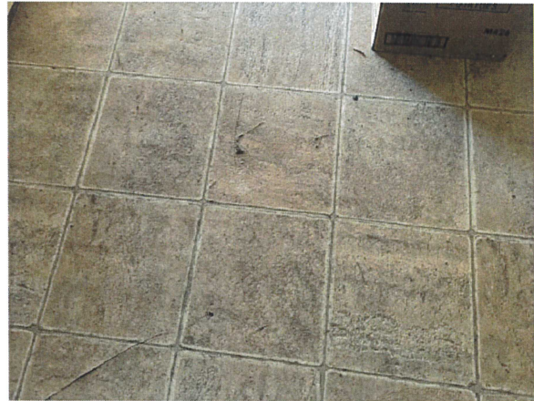
FAI-121-100223-001, 002, 003 None Detected, Brown Vinyl Sheet Flooring
